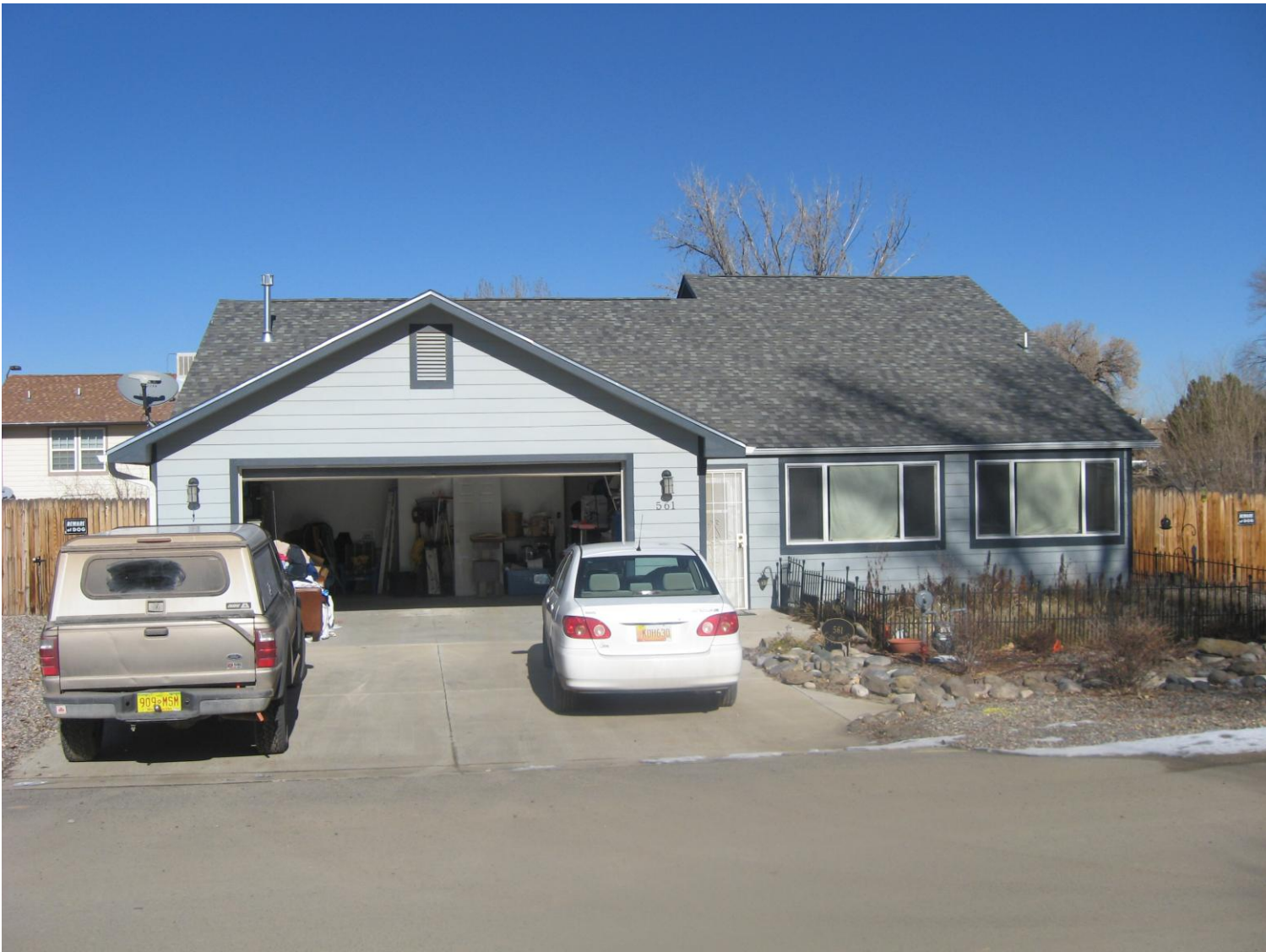
Front of house looking North
