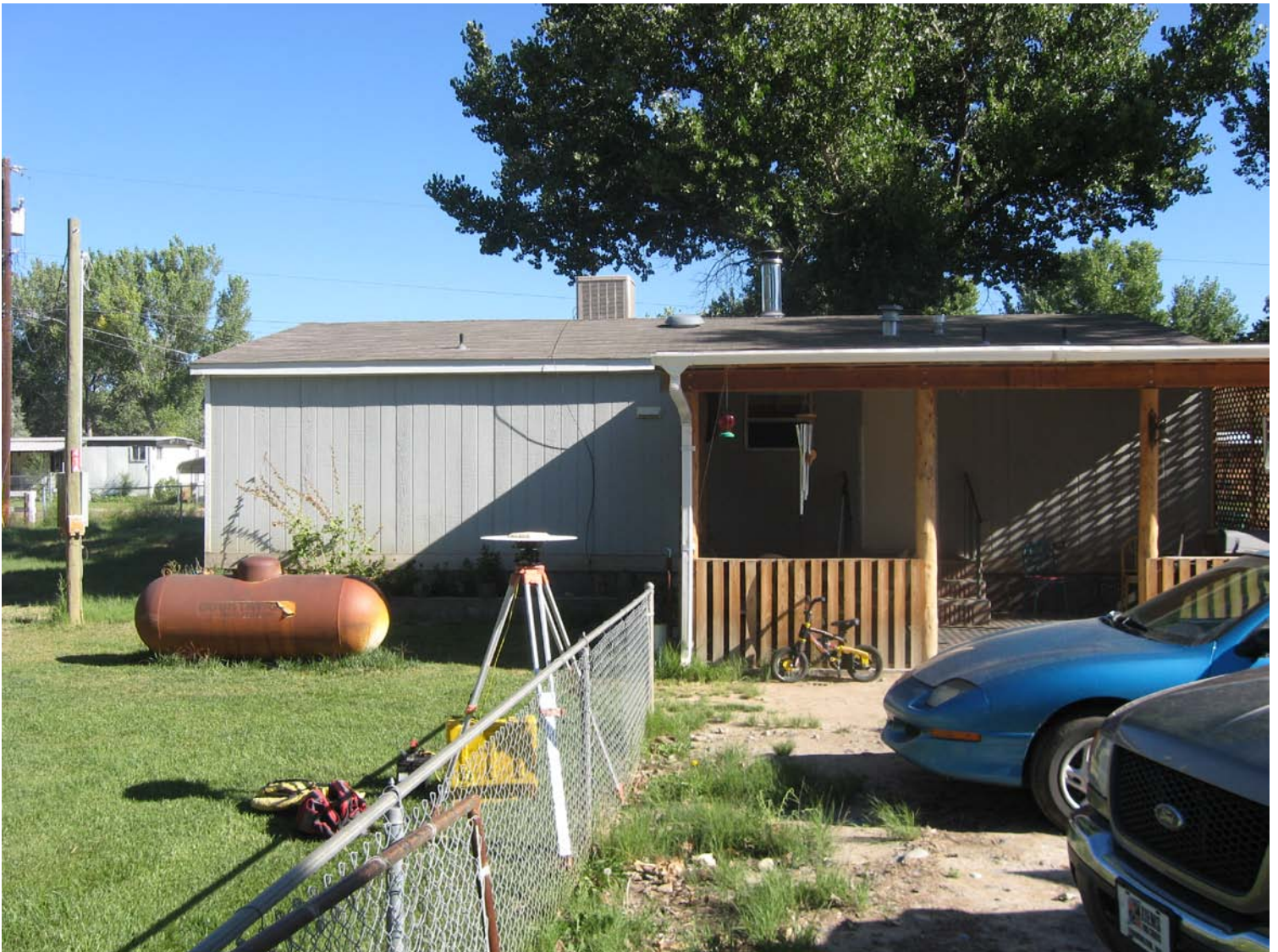
Front of House looking North
