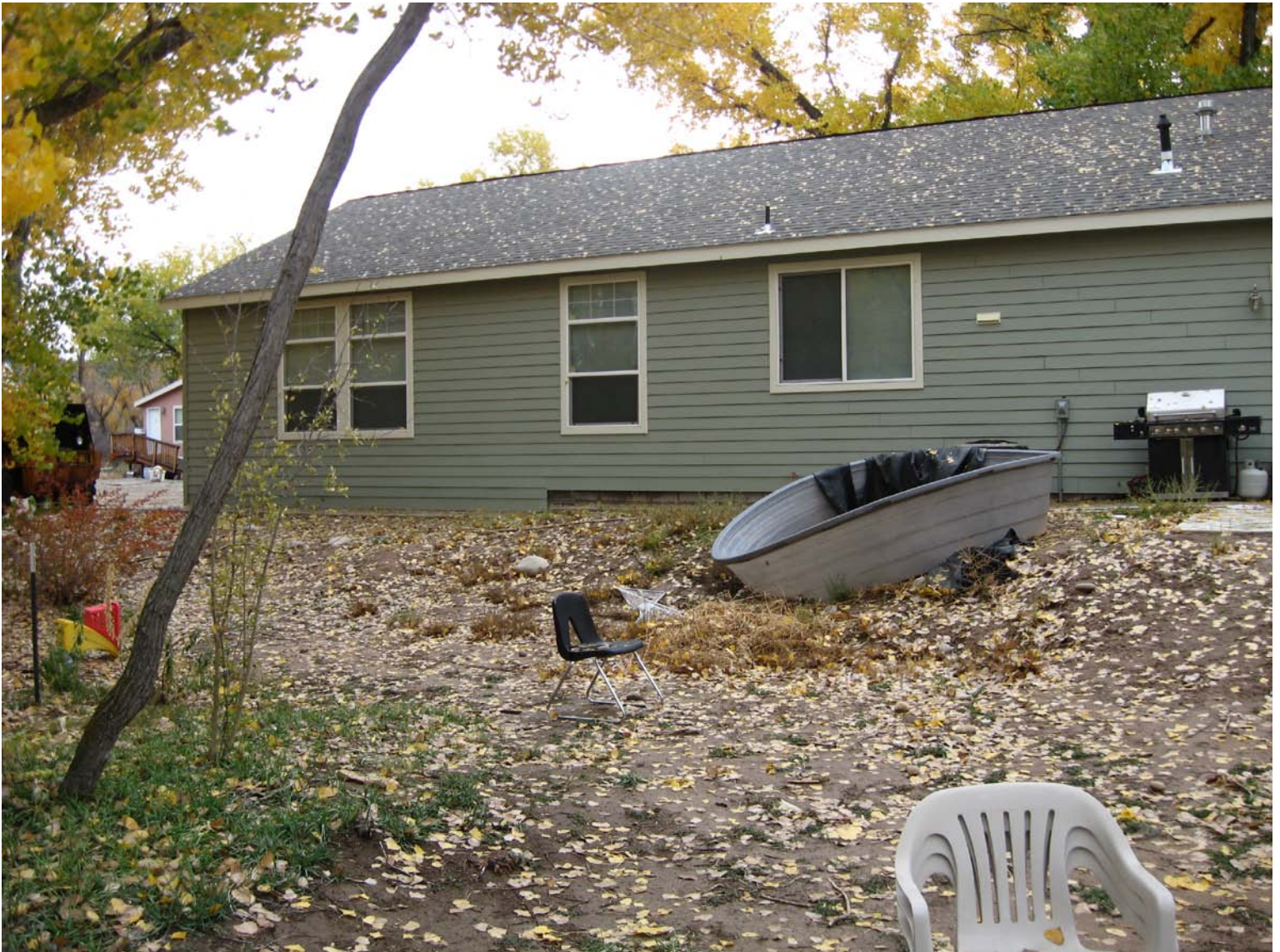
Back of structure looking East
