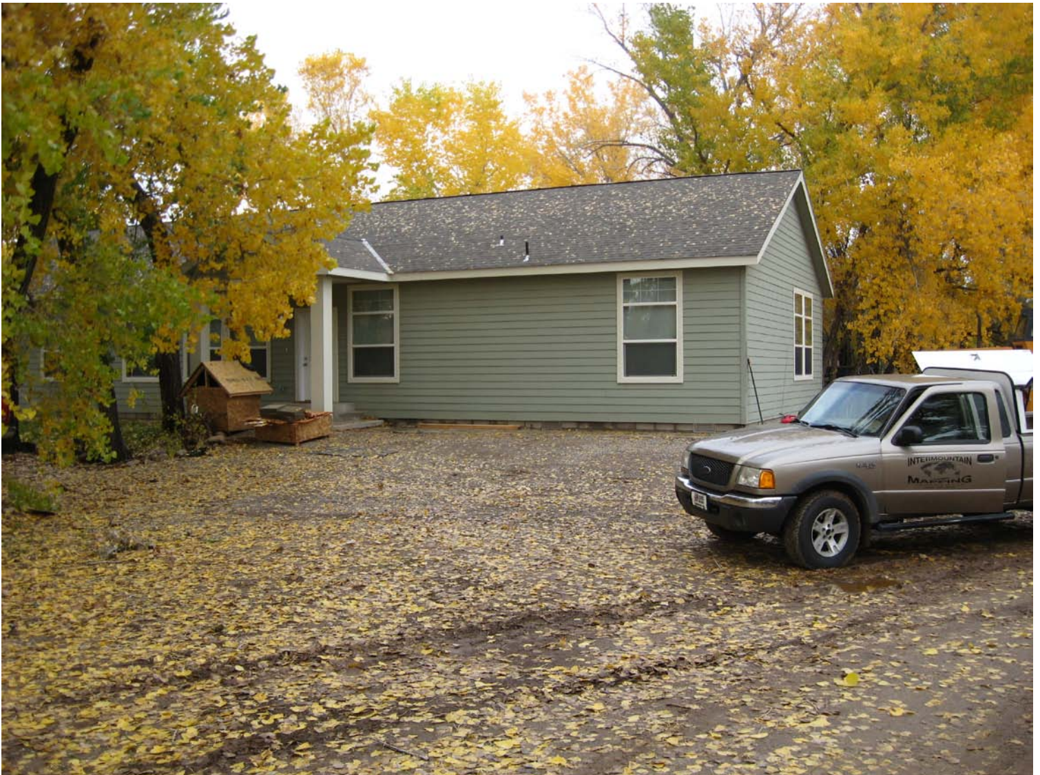
Front of structure looking West
